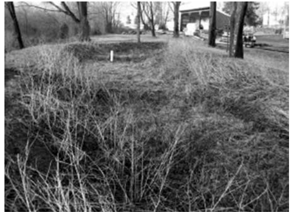
Complete and Vegetated Gravel Wetland
