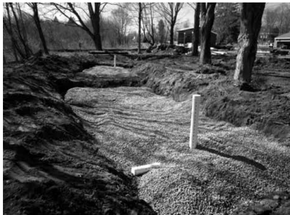
Excavated Treatment Cells Filled With Gravel
