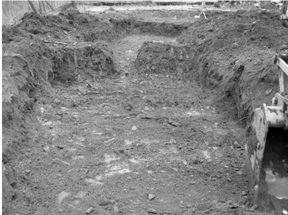
Excavated Treatment Cells Before Addition of Gravel
